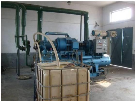
Refrigerator which needs cleaning, and cleaning equipment
