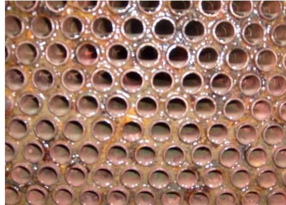
The cleaning effect is good, the tube sheet exposed metal color
