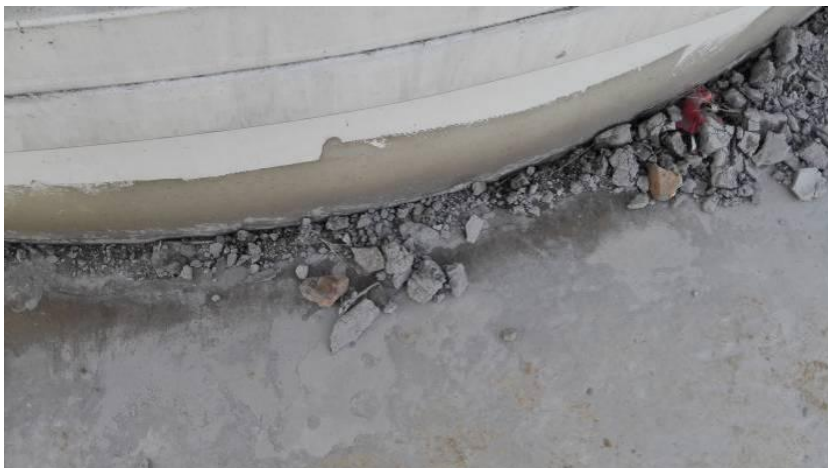
The Gap of External Loop \geq 2 mm
