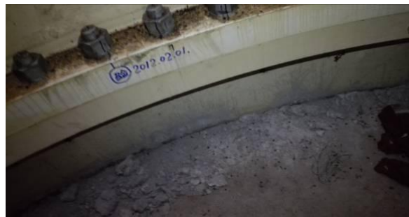
The Gap of Internal Loop \geq 2 mm
